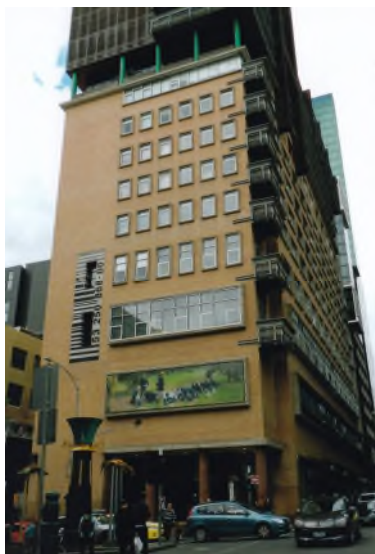
Former Russell Street Telephone Exchange (2017)
